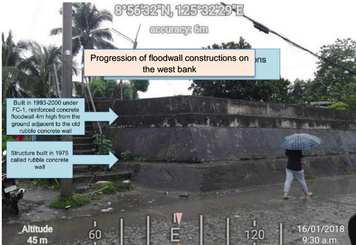
Figure 10. The FC-I floodwall on the west bank built beside the old concrete rubble wall.
