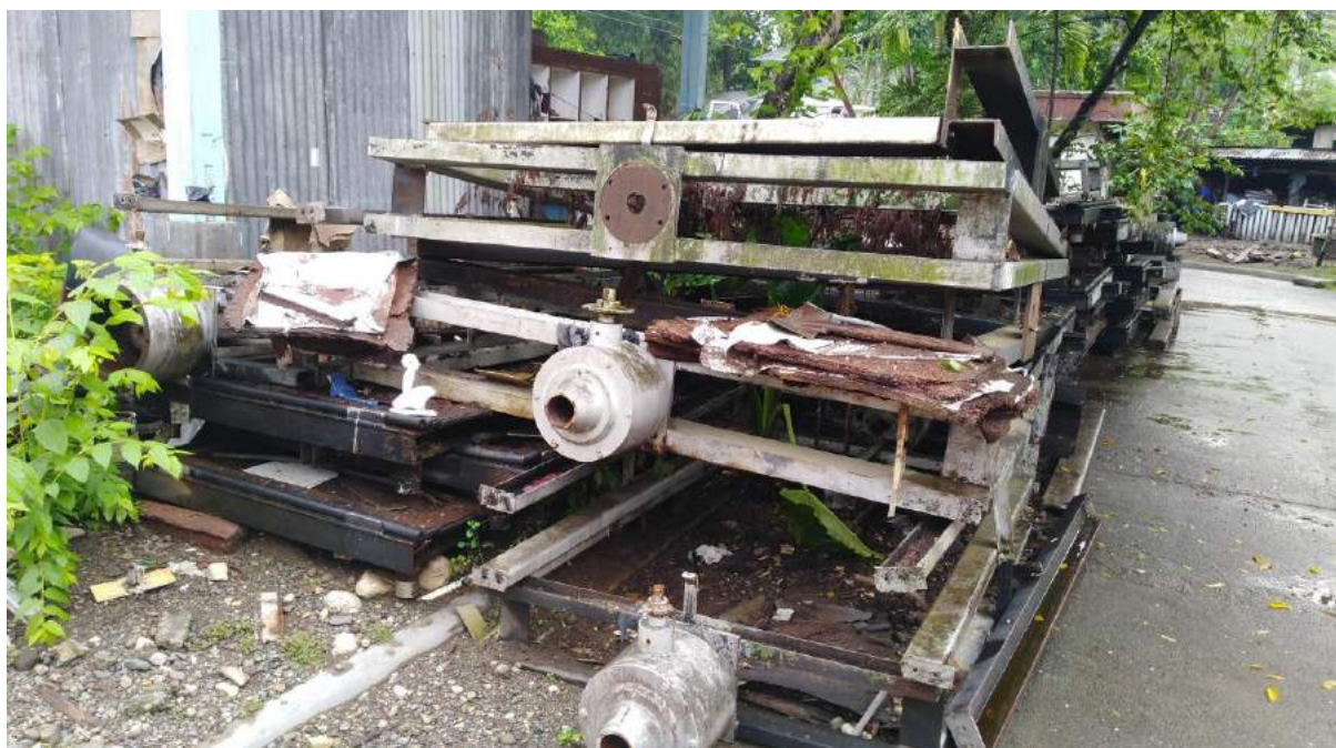
Figure 28. Recovered steel parts of the drainage sluice gates
