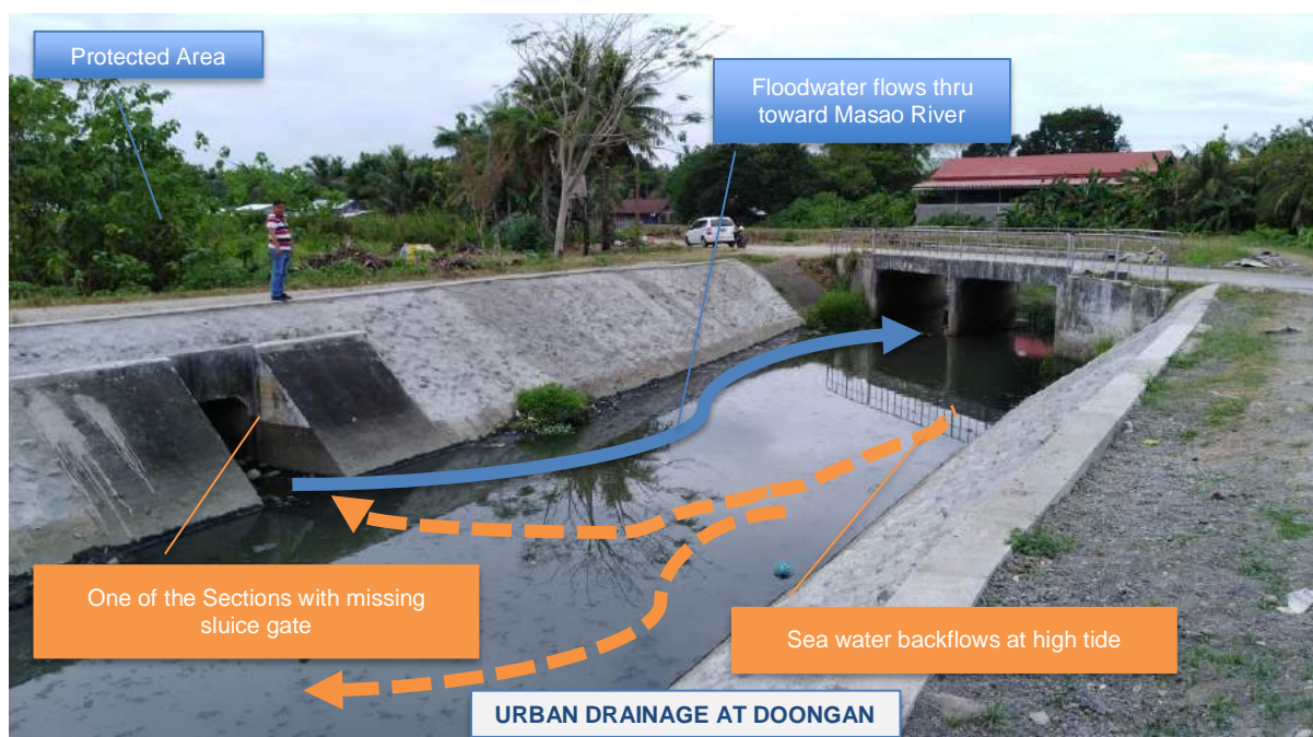
Figure 29. Missing Drainage Sluice at Doongan
